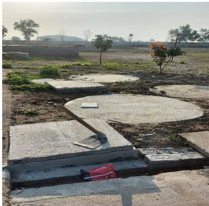
Leach Pit Rain water charging
